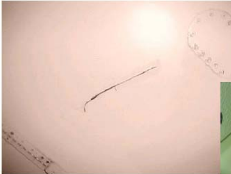
Visible damage on outside surface
