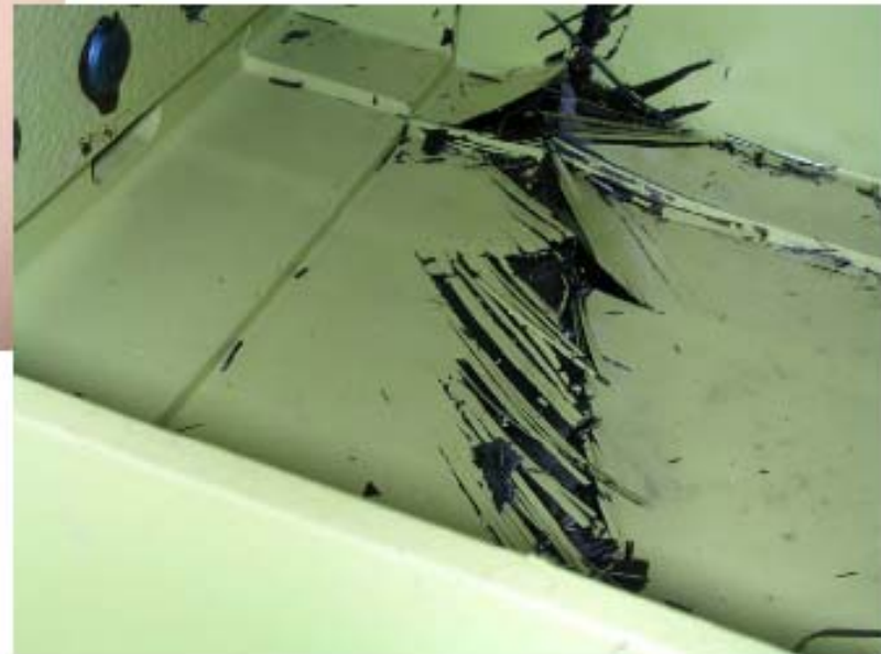
Total damage on inner side of structure
